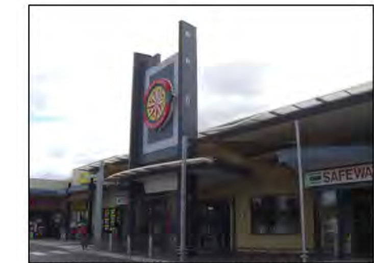
EXISTING MAIN ENTRANCE WEST ELEVATION
